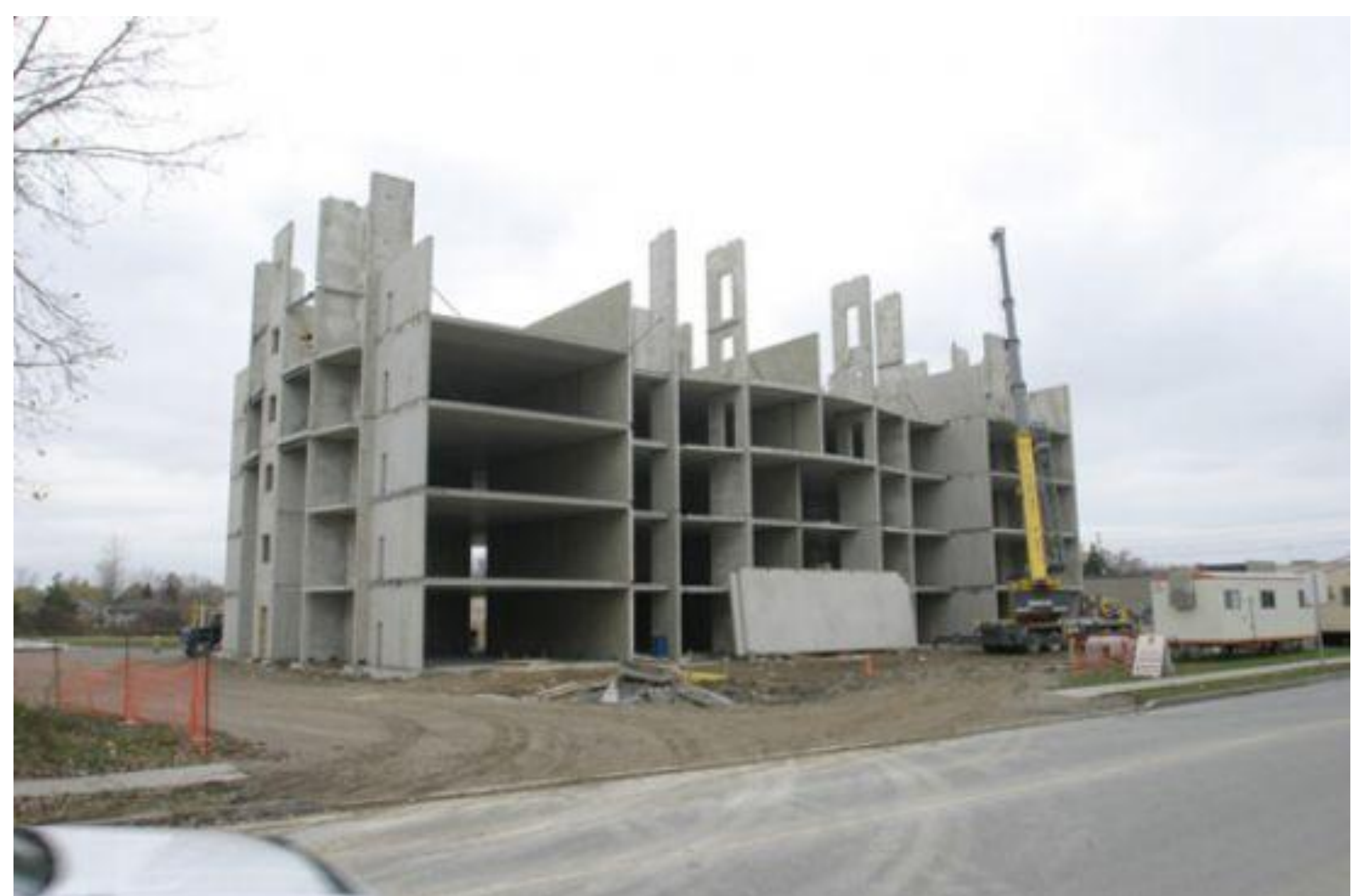
Figure 2: Assembly of Pre-cast Concrete (Erection)
