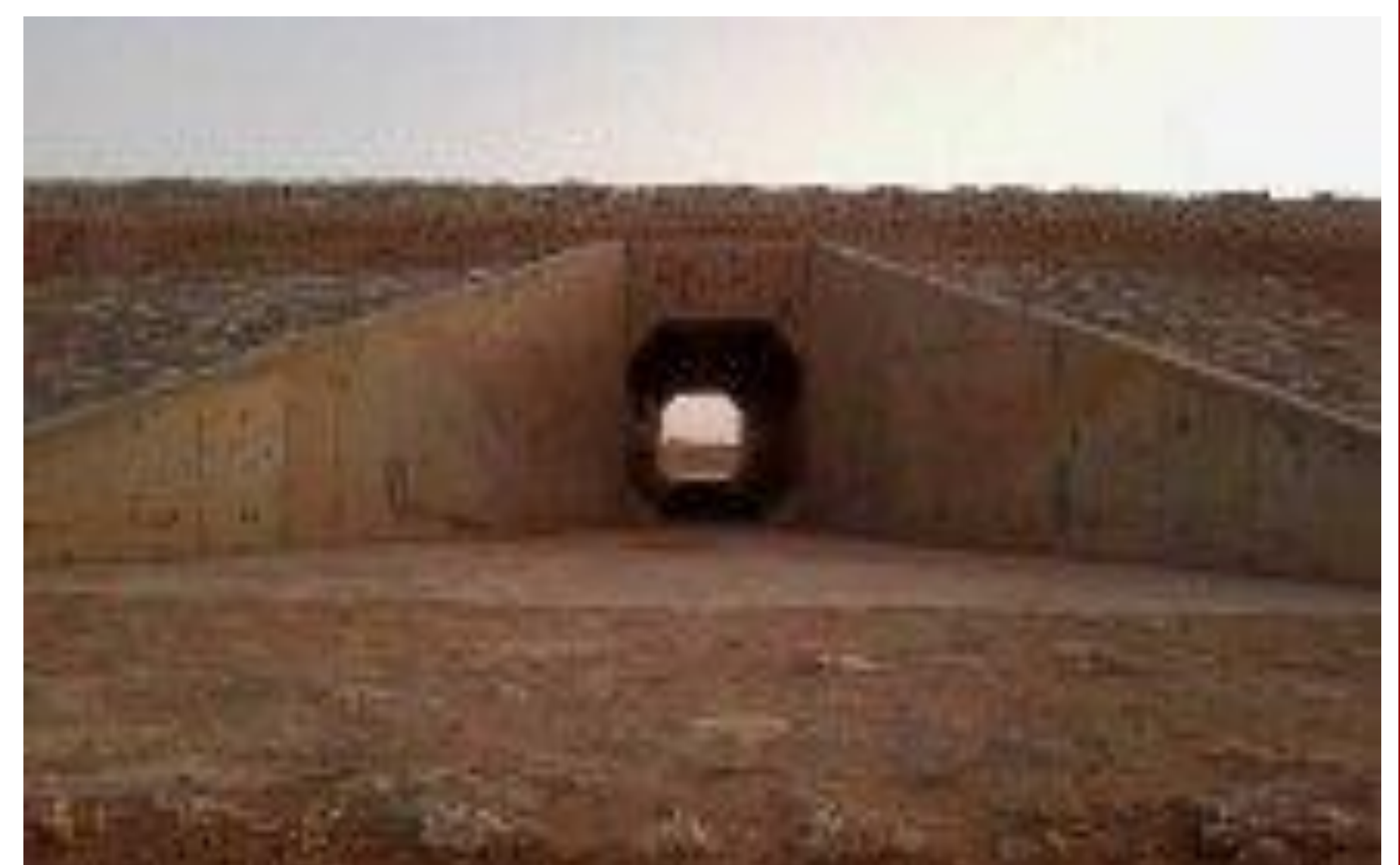
One vent box culvert
