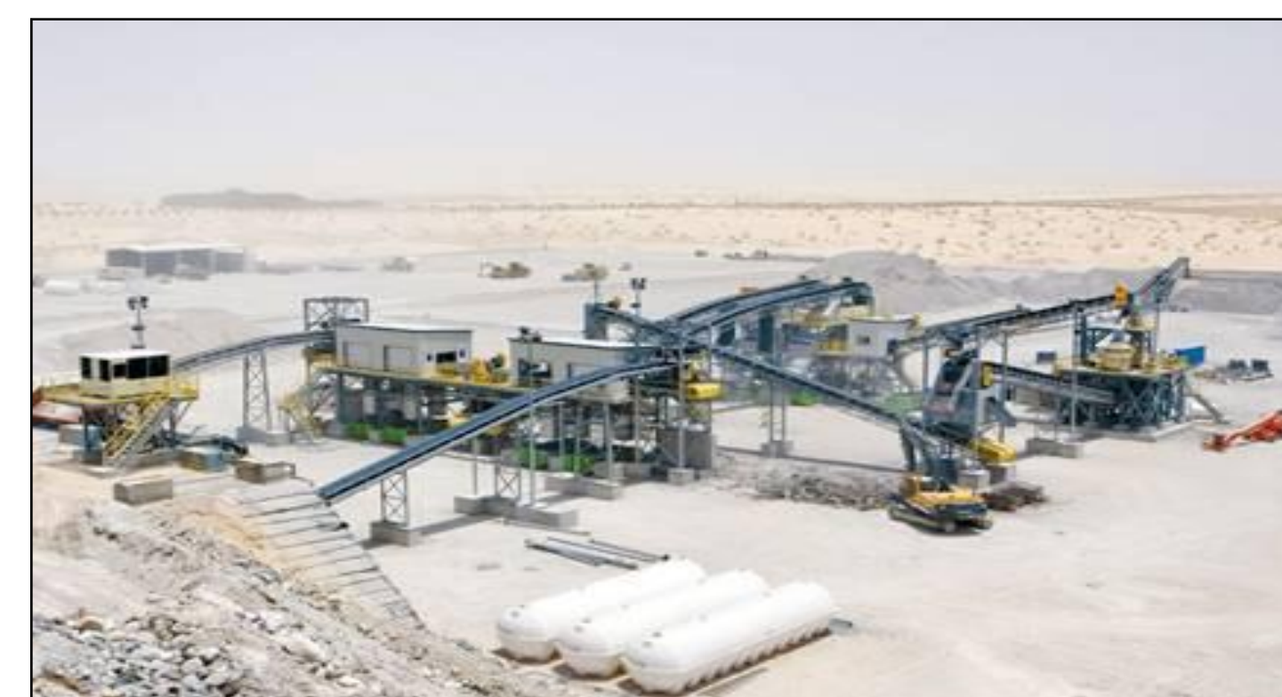
Example of a construction and demolition plant
