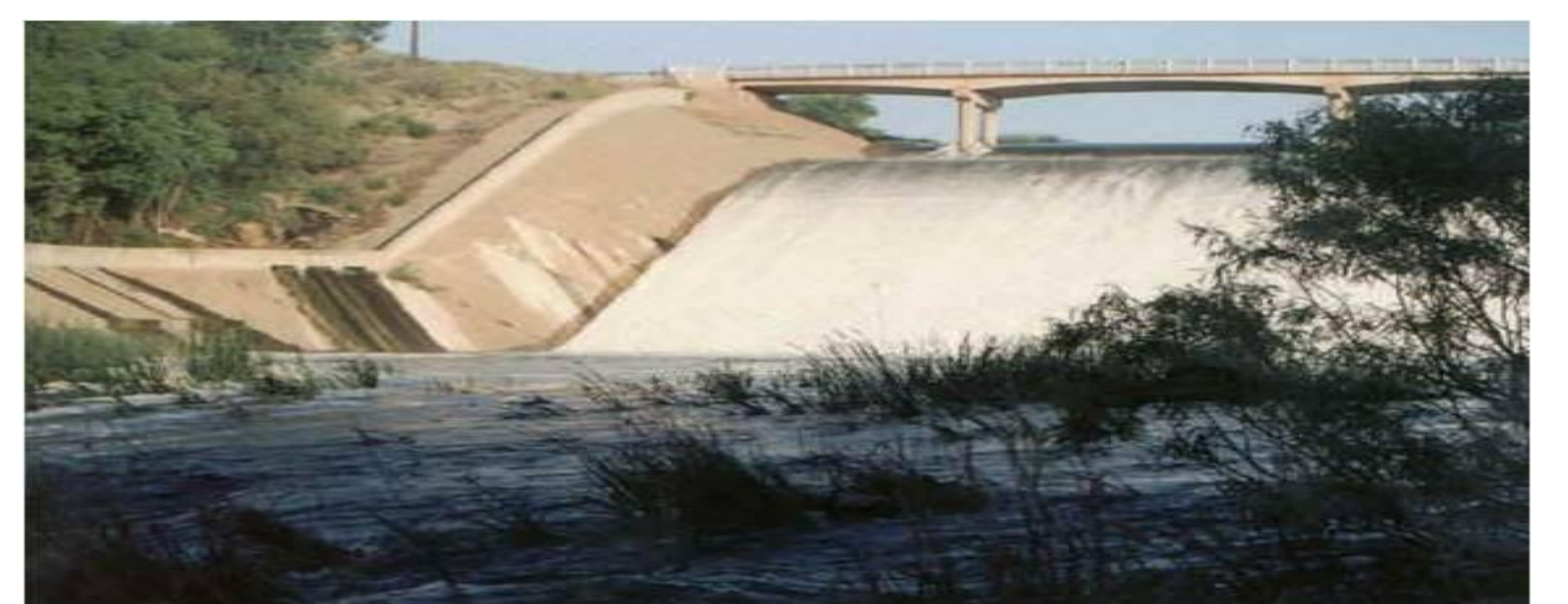
Dissipating water energy over the spillway
