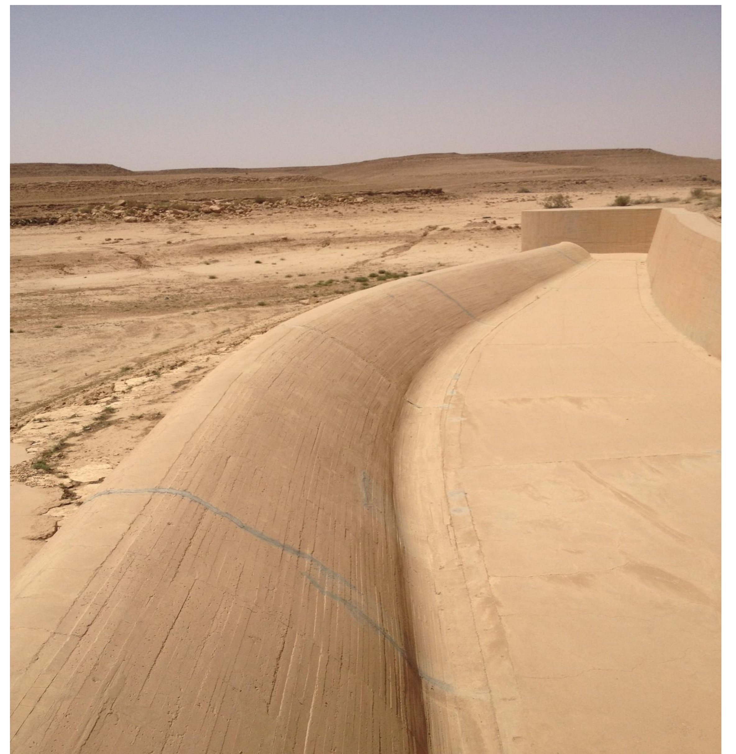
Majmaah dam Side Weir Spillway
